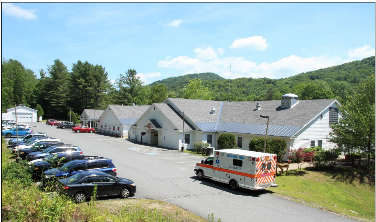
Grace Cottage Family Health & Hospital, Townshend, VT
