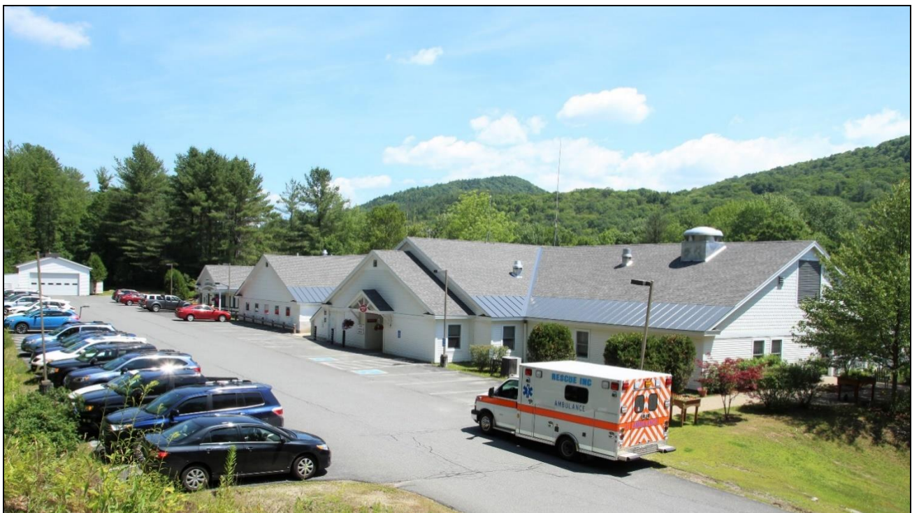
Grace Cottage Family Health & Hospital, Townshend, VT
