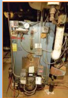
So long, antique boiler!
